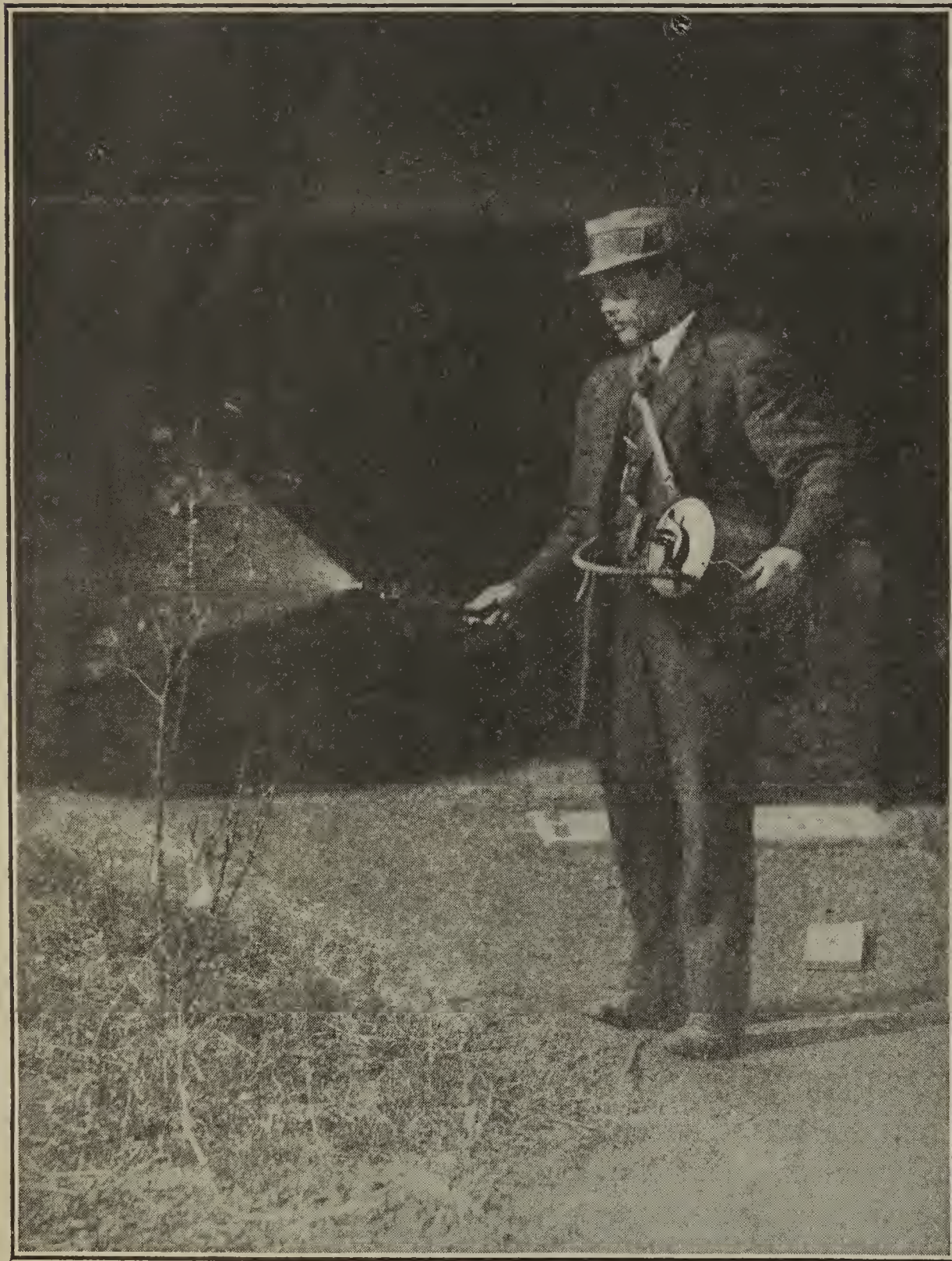
FIG. 2.—Spraying a rosebush with compressed-air sprayer. This is one of the best types of small sprayers for garden use. Prices range from $5 to $8.50, depending upon whether the tank is made of galvanized iron or brass.
